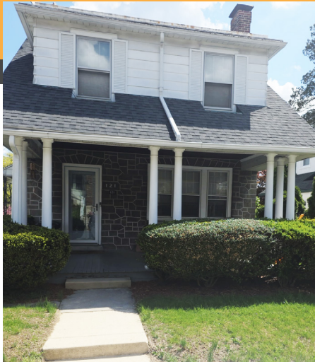
Front of Willard's home with new windows.
