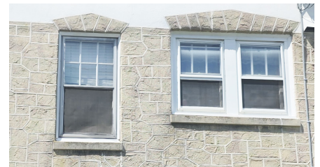
Brand new windows installed in Willard's home.
