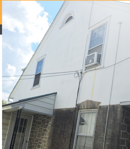
Back of Willard's home with new windows.
